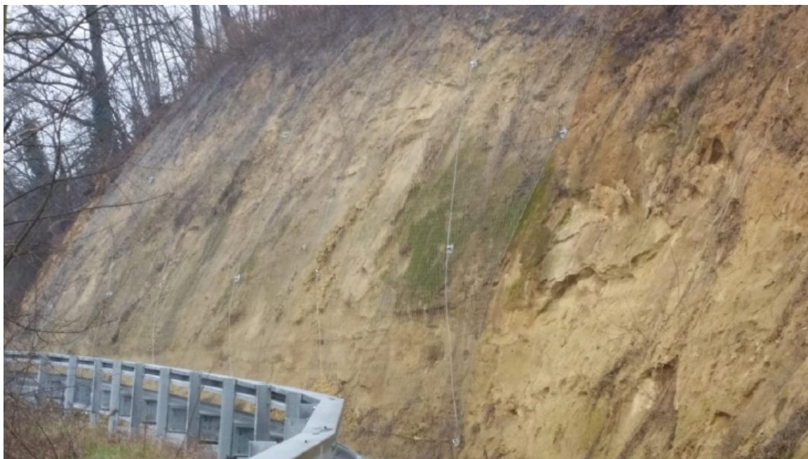
Figure 1. Metal mesh containment adhering to the Sabbie di Asti outcrops to mitigate the risk of falls on the viability.
